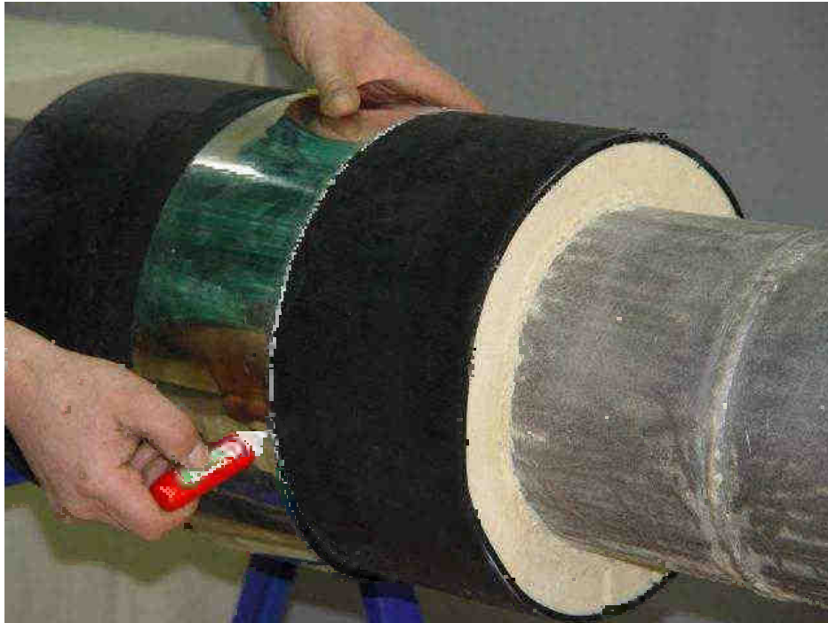
Photo 28 Tracing the location of the external edges of the heat shrinkable sleeve
