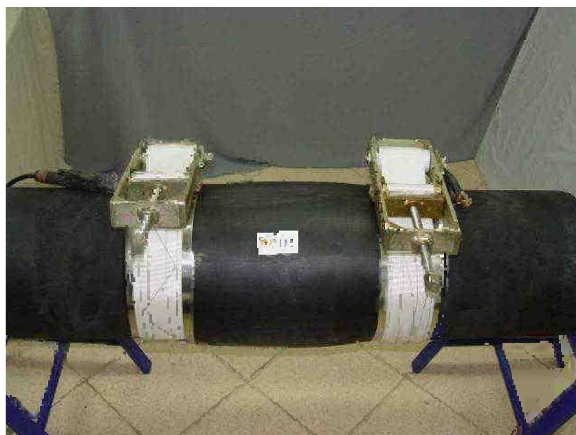
Photo 47 A view of a heat shrinkable, metal separator tightened together with a belt fastener ready for welding operation
