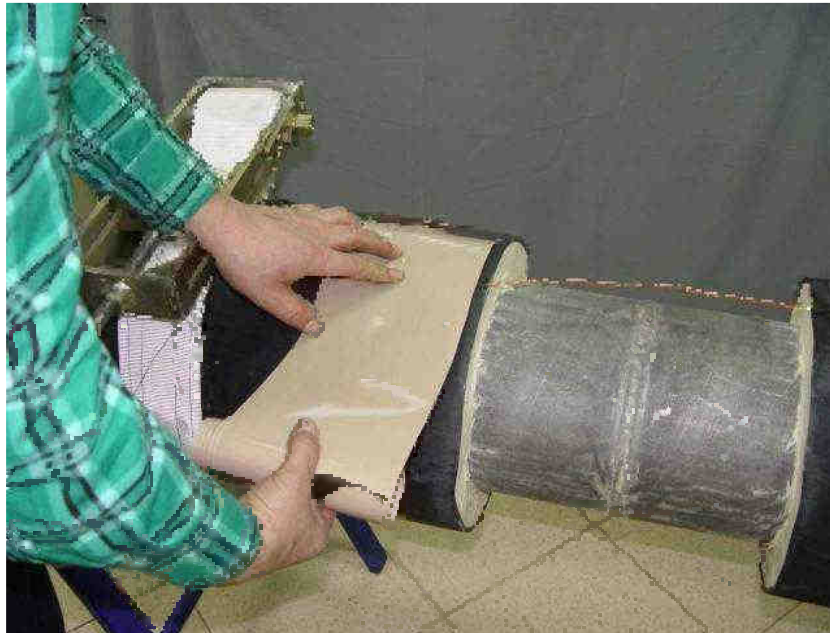
Photo 38 The heating elements wrapped in a teflon foil
