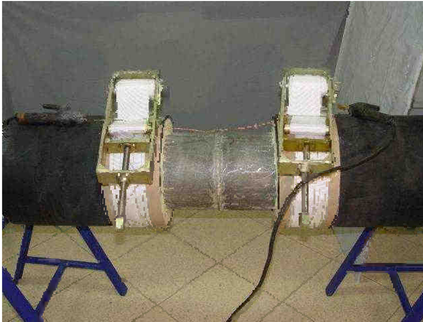
Photo 40 Terminals connected with the heating element wires
