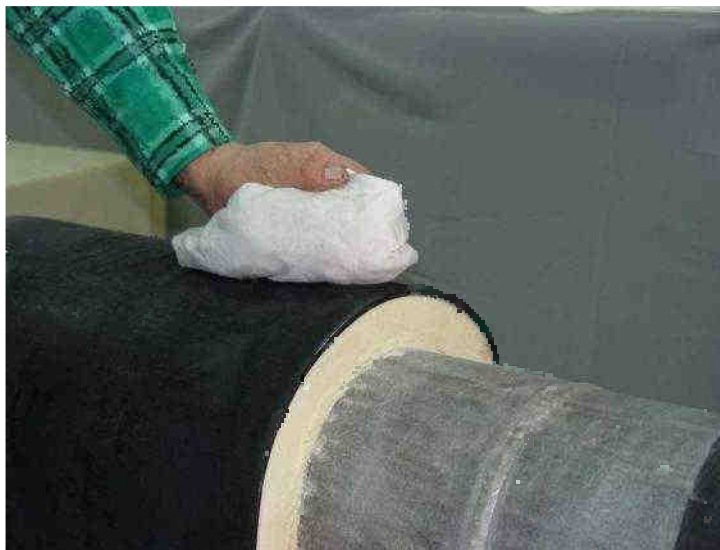
Photo 26 Cleanin the casing pipe of a preinsulated element with acetone
