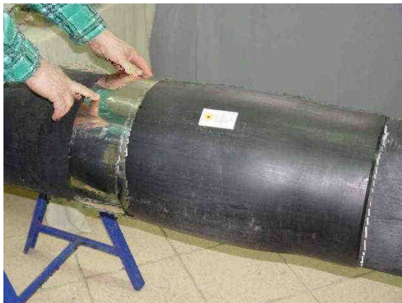
Photo 54 A heat shrinkable sleeve and a metal separator
