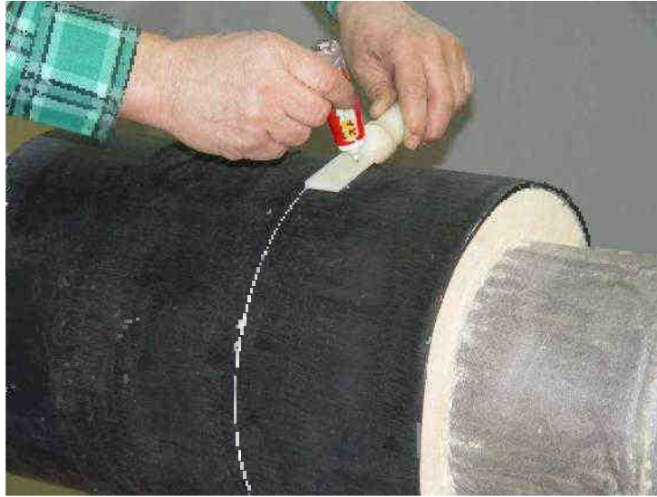
Photo 29 Tracing the location of the heating tape
