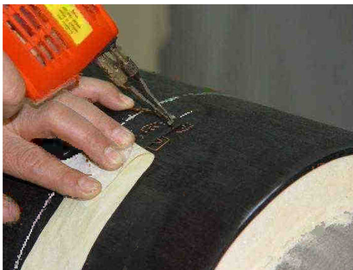
Photo 30 A heating element is fixed to the casing pipe by means of a hot soldering gun tip while the adhesive is gradually detached
