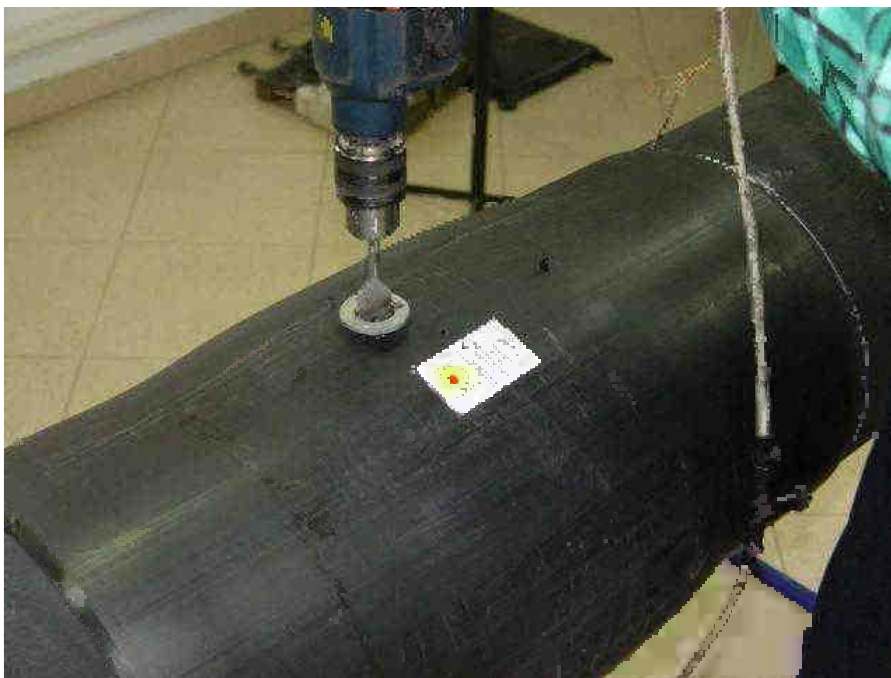
Photo 48 A 25 mm hole drilled with a flat drill and drilling machine
