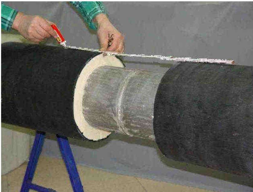
Photo 27 Marking the calculated dimensions in tracing the location of the edge of the heat shrinkable sleeve
