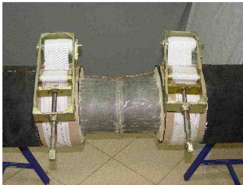
Photo 39 Placing clamp belts over the heating elements wrapped in a teflon foil
