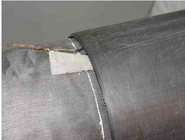
Photo 42 A detail – inserting aluminium wedges
