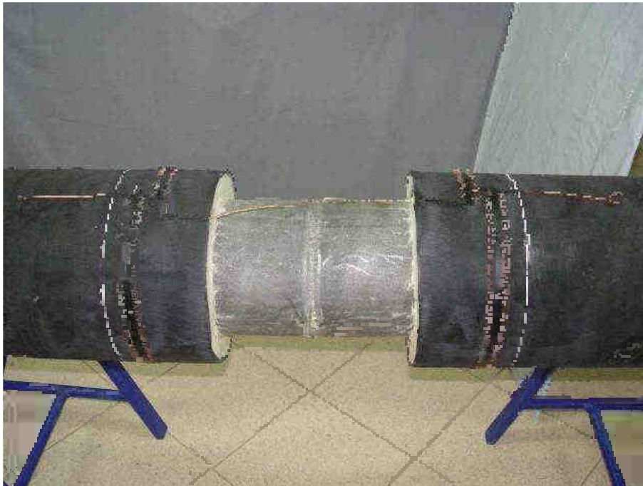
Photo 37 Copper wires of the heating elements connected
