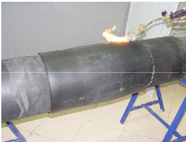
Photo 43 Shrinking a heat shrinkable sleeve ends with a soft flame from an LPG burner
