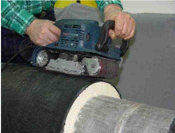
Photo 25 Cleaning casing pipe of a preinsulated element with a hand held electric belt grinder
