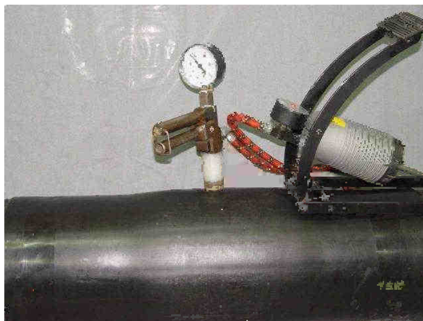
Photo 50 A joint being filled up with air
