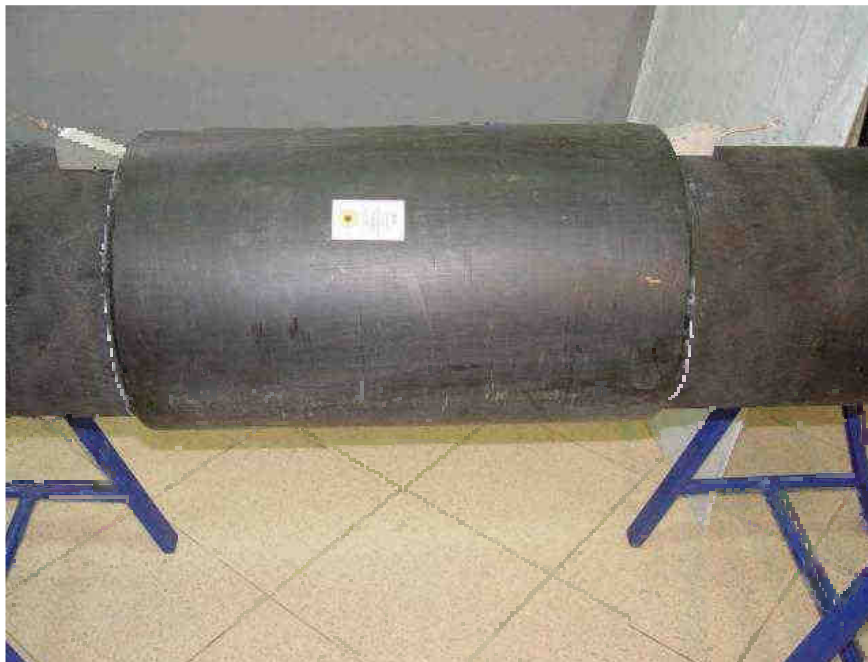
Photo 41 The manner in which a heat shrinkable sleeve has to be propped with wedges before the sleeve starts being shrunk
